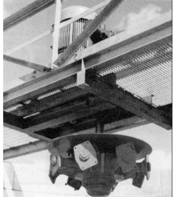
Figure 3 Electrically Operated Variable Pitch Fan
