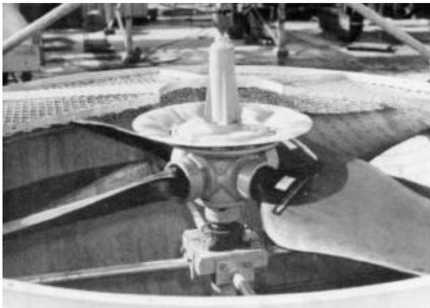
Figure 1 Typical Variable Pitch Fan
