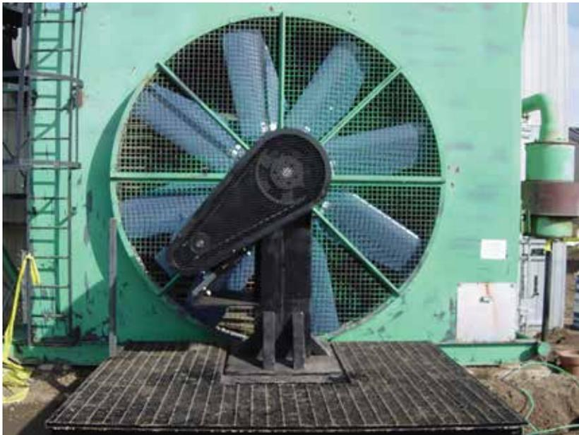
Here's a totally converted and engineered system that we can provide. This was originally a left-hand, low-efficiency fan, V-belt driven off the engine jack shaft. Now it's a VFD/motor/timing belt package with a right-hand, high-efficiency fan. Since it runs independently, the fan doesn't draw load off the engine. This is ideal for many obvious reasons like preventing winter freeze-up issues, saving on engine fuel, cooling better at lower engine speeds, and lowering noise levels.
