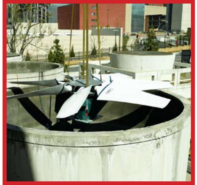
The result of the research and development is the Baldor•Reliance RPM AC Cooling Tower Direct Drive Motor, which features a power dense, laminated steel, finned-frame construction. A proprietary Permanent Magnet Rotor (PMR) design using high-flux magnets allows the motor to be manufactured in a compact form, similar to the gearbox it replaces.
