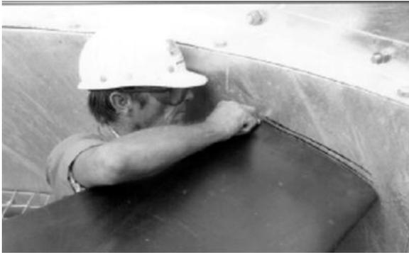
Trace each blade with marker onto plenum.
