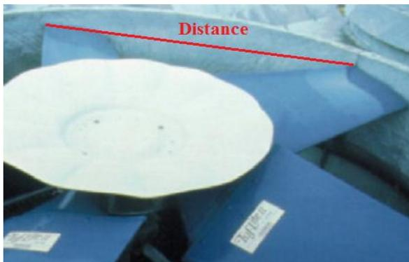
Measure From trailing edge to trailing edge of the next blade. All sweep measurements must be within 1" of each other.
