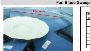
Measure From trailing edge to trailing edge of the next blade. All sweep measurements must be within 1" of each other.
