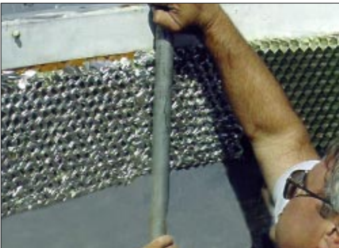
Figure 6 - Rolling Section Using Pipe
