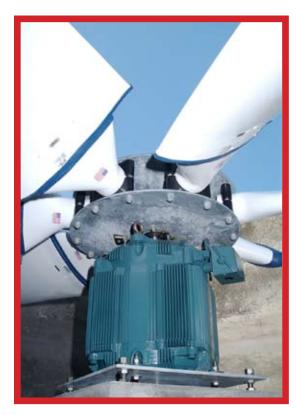
The combination of these innovative technologies has allowed the company to build a high torque, low profile motor, with the fan mounted directly on the motor shaft. It's a synchronous machine that runs at precise speeds without slip in combination with a Baldor Permanent Magnet Cooling Tower drive.
