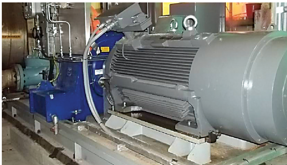
To the left is the old steam turbine coupled to the pump. The picture above shows the after picture, with the electric motor direct coupled via disc couplings to the Voith Turbo variable speed drive which is directly coupled with another spacer disc coupling to the pump.
