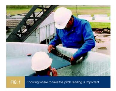
**Pitch.** Always know and record the pitch for all fans. Every blade (for each particular fan) needs to be at the same pitch ( $\pm 0.5^{\circ}$ ). It is also very important to know exactly where to take this pitch reading (Fig. 1). Most ACHE manufacturers have excellent Websites. This, and additional information including maintenance manuals and fan
