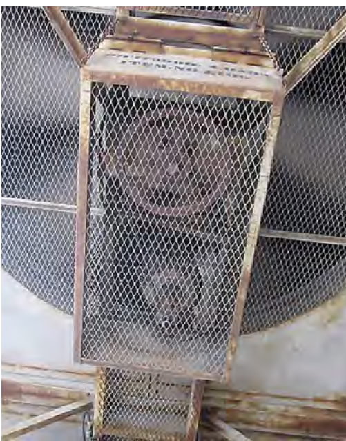
Left: View of belt drive under larger air cooler fan
