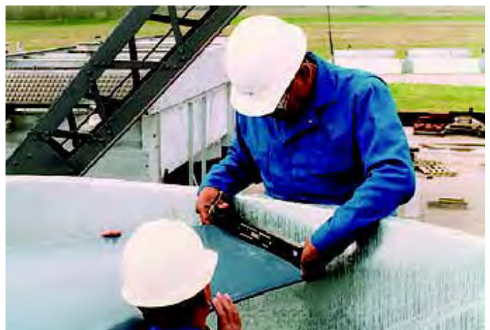
FIG. 1 Knowing where to take the pitch reading is important.
