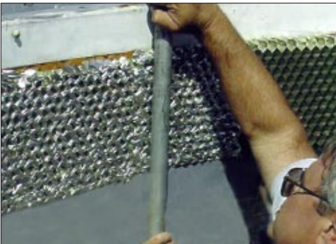
Figure 6 - Rolling Section Using Pipe
