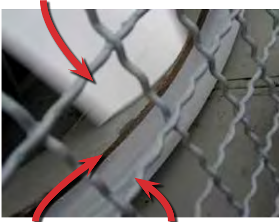
Fan-ring extension for low-noise project
