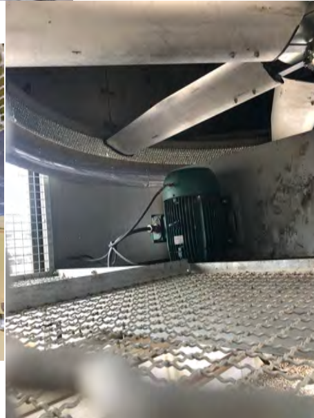
Elliptical Inlet Bell 0.10D/0.15D
