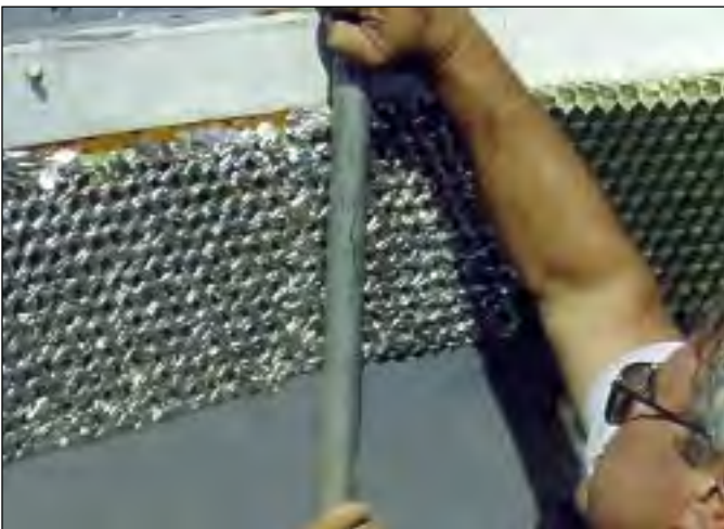
Figure 6 - Rolling Section Using Pipe
