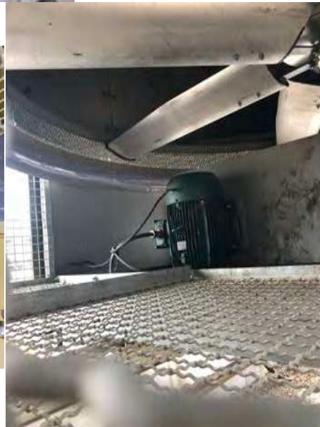
Elliptical Inlet Bell 0.10D/0.15D
